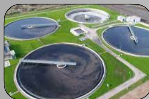
PURIFICATION OF WASTEWATER
